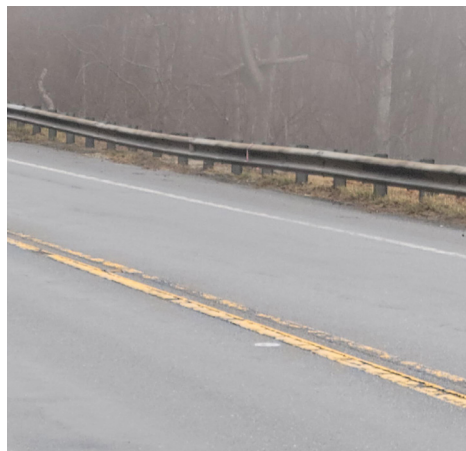
Guardrails will be repaired and improved
