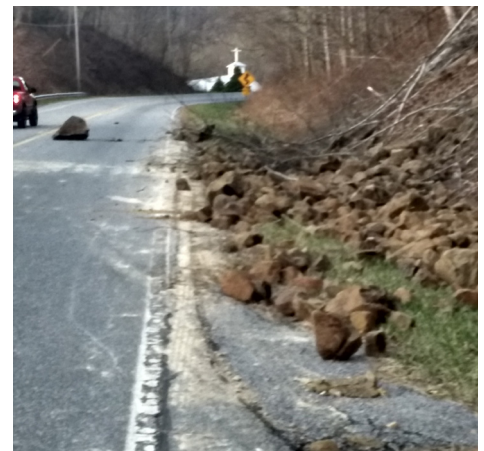
Slopes and soil stability will be improved
